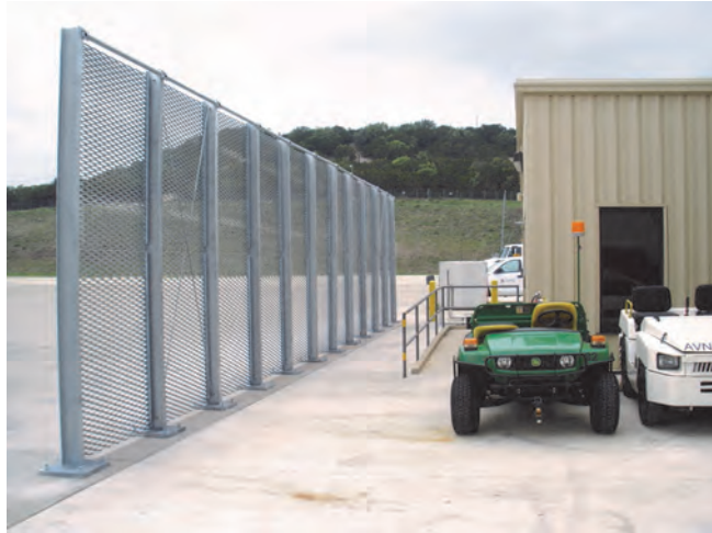
Vertical JBS protecting ground support equipment and structures
